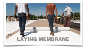
Laying the new membrane and heat sealing all edges and around all protrusions is the final step. To assure your roof is not exposed during the entire project, we repeat all steps for each section.
