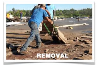
Removing the deteriorated roofing material and insulation requires extracting screws, cutting into manageable sections and hauling away. Many times the insulation is water logged and simply disintegrates.
