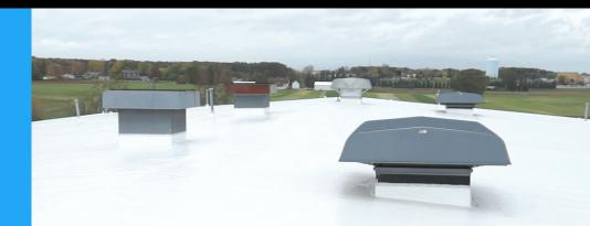
White is the only single-ply membrane rated by the EPA *Energy Star*<sup>®</sup> roof products program. Even after three years of exposure, it retains more than 86% reflectivity.
